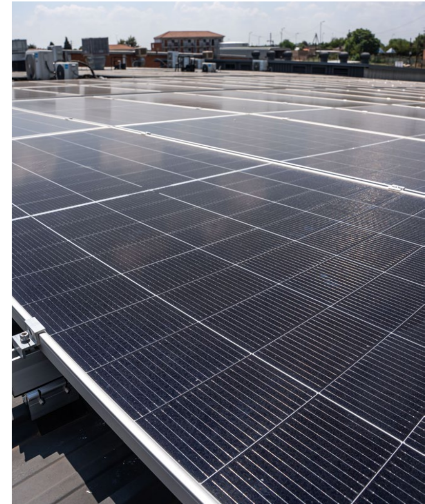
TOP: Renbro Centre BELOW: Phoenix Plaza
